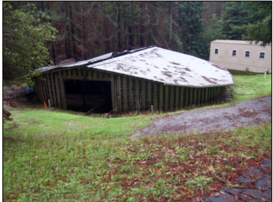
The park's wastewater treatment plant survived the fire unscathed. Whether or not it will ever be used again will be decided in the coming years
